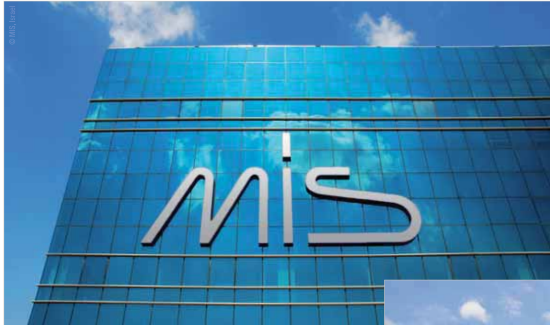
• MIS Firmenzentrale. • MIS headquarters.
